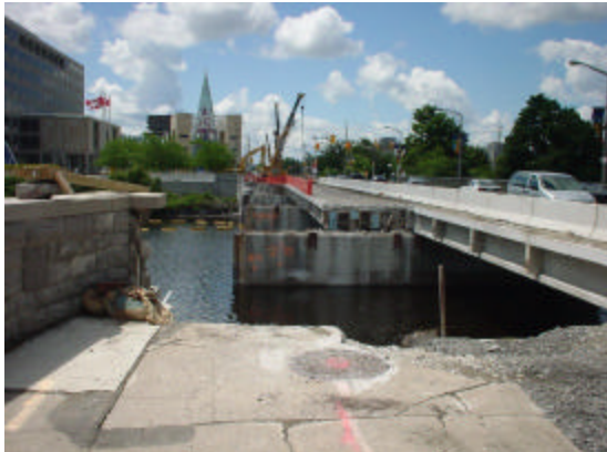
Removal of old bridge deck
