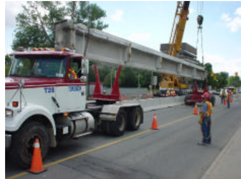
Loading truck with removed beam
